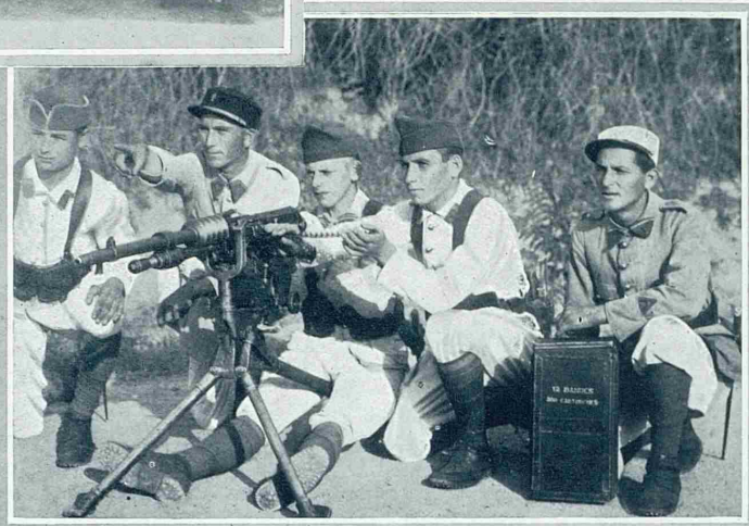
COVER FOR THE WORKERS: One of the 1914 model Hotchkiss machine-guns which are used to protect the labouring parties
